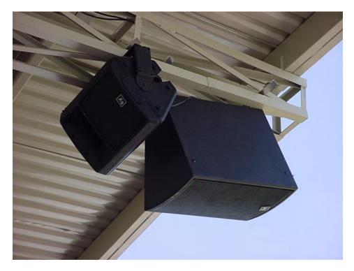
Thanks to the calculations carried out by Enrique Lask (Sales Representative for Electro-Voice in Mexico), the result was a more uniform SPL distribution and better coverage between loudspeakers. The distribution was designed in accordance to the coverage standard of the loudspeakers (FRi-152: 60 x 40 degrees, Sx100+: 60 x 60 degrees).
